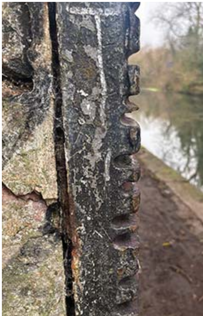
Broadwater Lane Bridge, with rope-eroded iron
