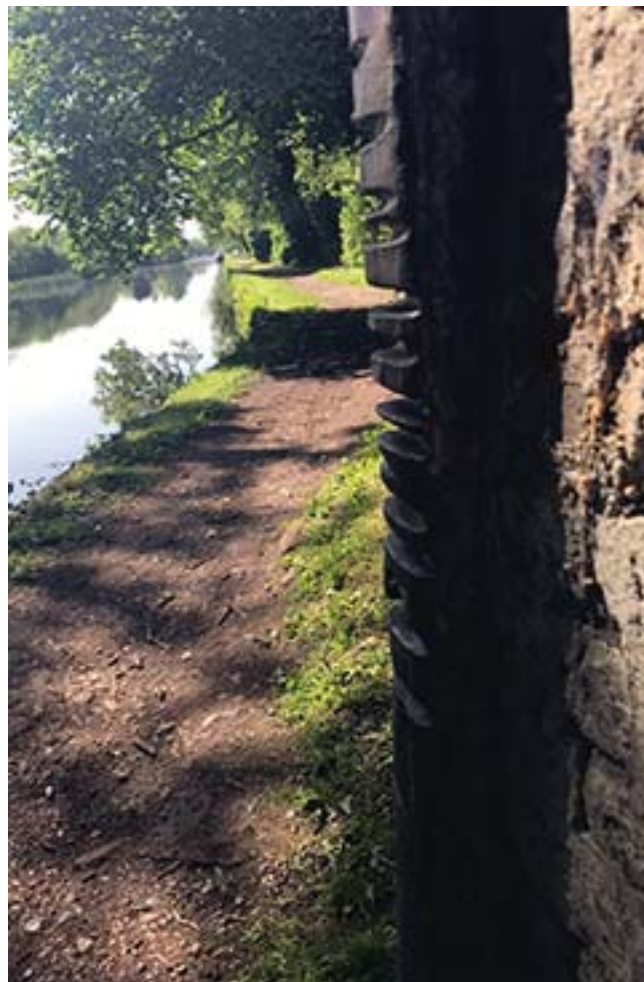
Broadwater Lane Bridge, with rope-eroded iron
