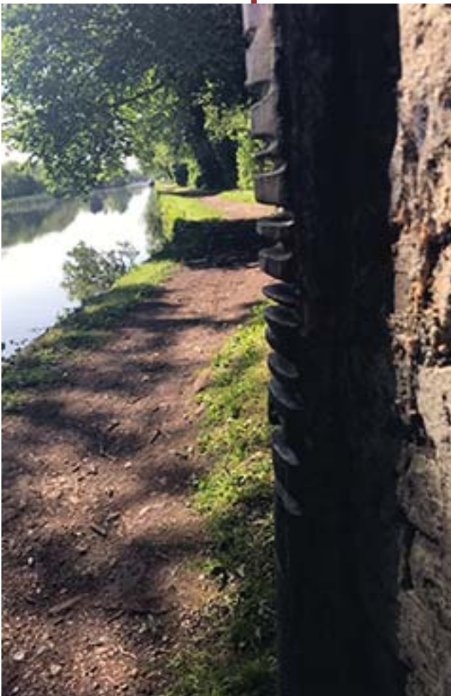
Broadwater Lane Bridge, with rope-eroded iron
