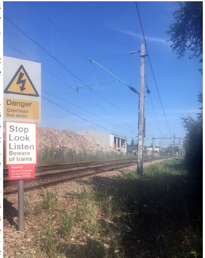
Railway crossing near Pitsea
